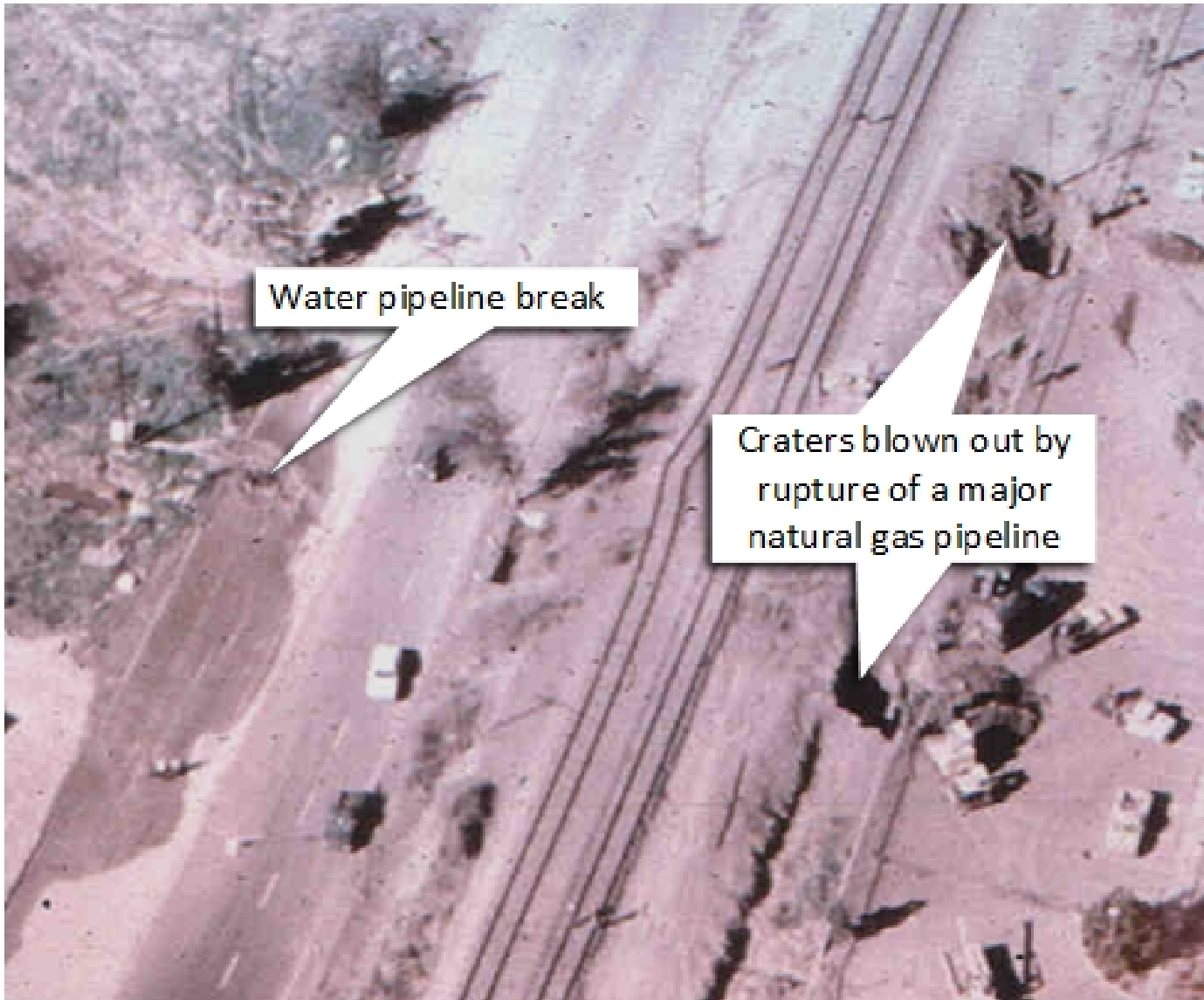
Fig. S8. Aerial photograph of localities of pipeline damage in front of SFJH (T.L. Youd photo)
