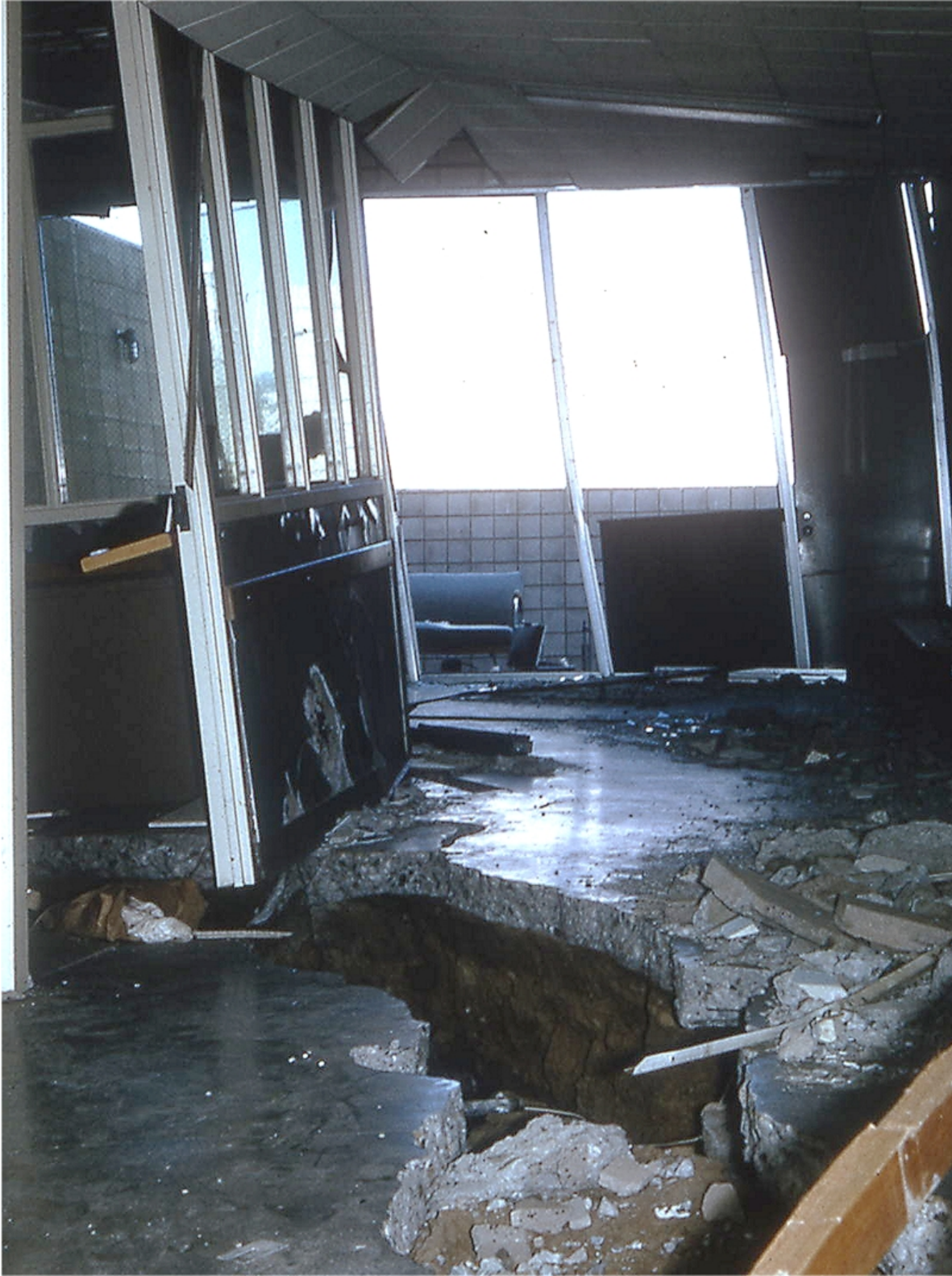
Fig. S6. Segment of floor slab pulled apart by extensional ground displacement beneath a SFJH building due to lateral spread movement (T.L. Youd photo)
