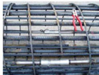
Reinforcing bars instrumented with stress meters
