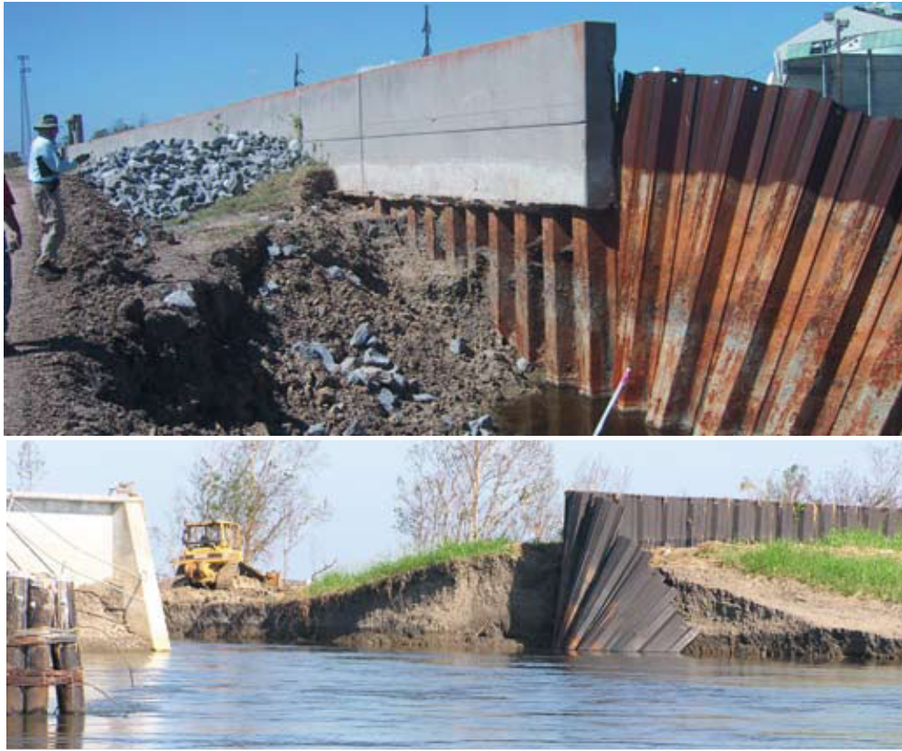
Figure 8.3 Failed I-Wall and Levee Sections
