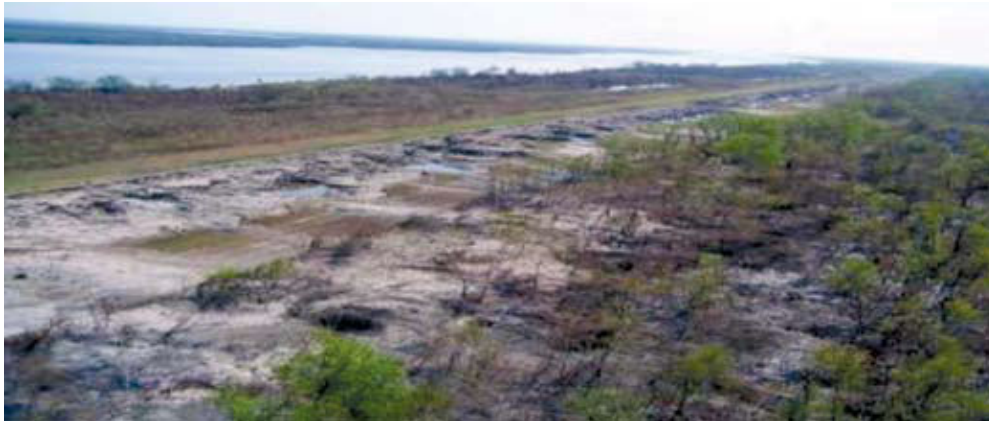
Figure 7.12 Obliterated Levee along the Mississippi River-Gulf Outlet
