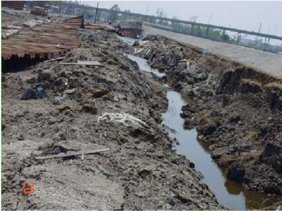
Figure 7.9 Industrial Canal East Bank South Failed I-wall
