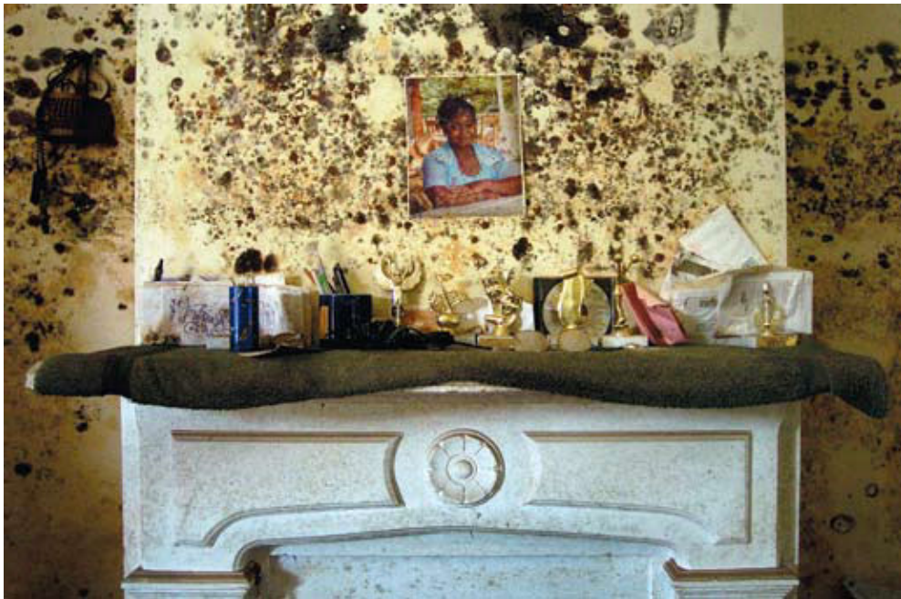
Figure 6.10 Overrun by Mold
