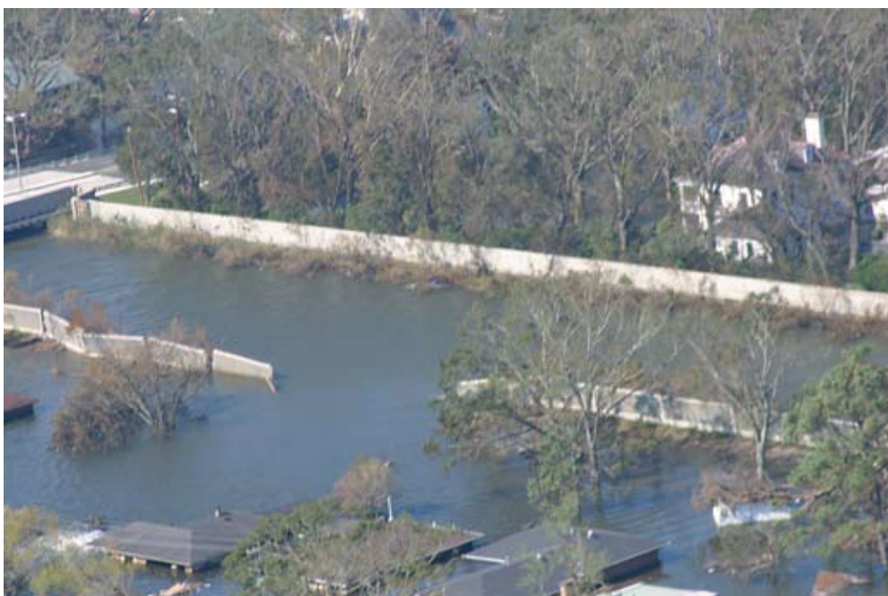
Figure 5.6 London Avenue Canal South Breach
