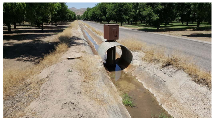
Fig. 7. Circular flume installed in a vineyard in Australia (image by author)
