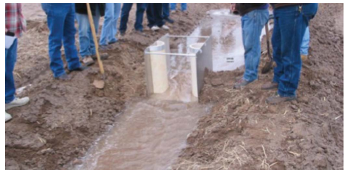
Fig. 5. Rectangular flume installed in an unlined ditch in southern New Mexico (image by author)
